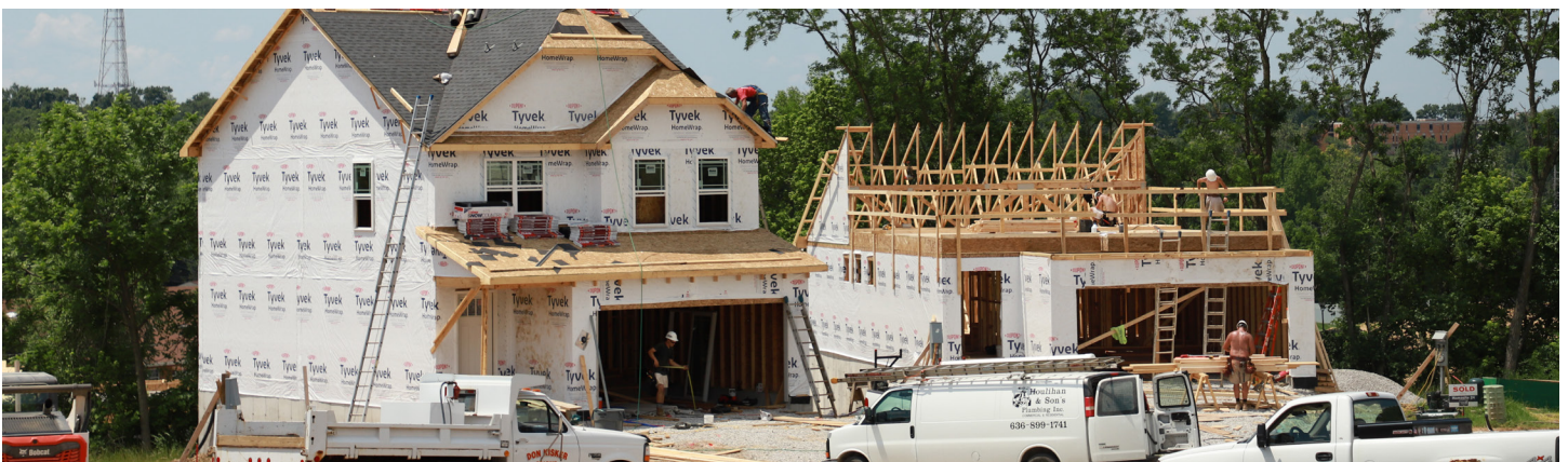
New housing construction in Maryland Heights
