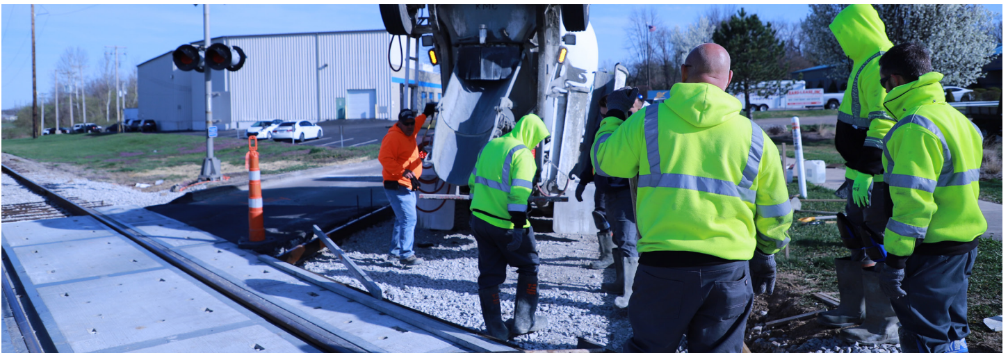
The Department of Public Works replaces concrete at a railroad crossing.
